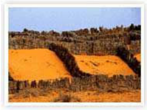
establishment of strips of artificial dunes with palm-leafs
